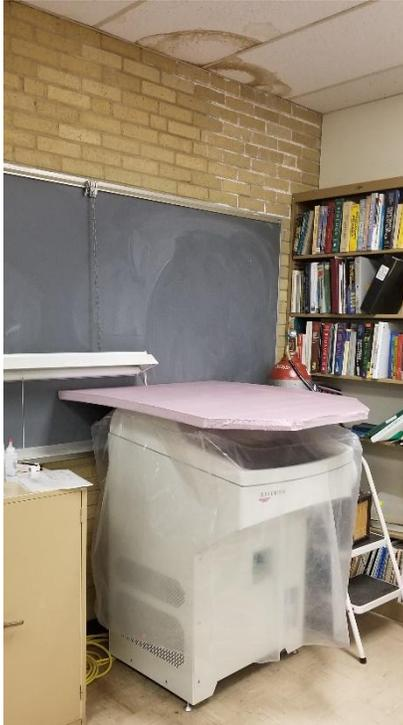
*Water leak above cryostat (laboratory equipment)*
