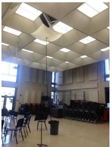
Ceiling leak (with improvised drainage system)
