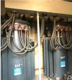
*Transformer from the 1950s* (with exposed live copper)
