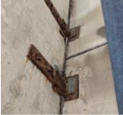
Rusted brackets, concrete pulling away
