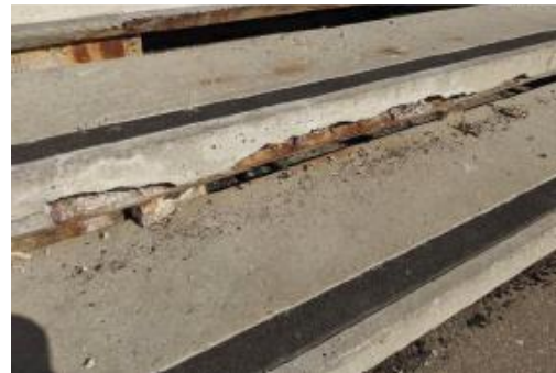
Damaged entry stair tread
