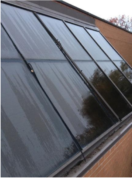
Aluminum cap damage & gasket popping out
