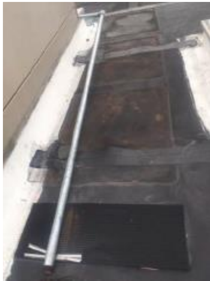
Deteriorating roof patches
