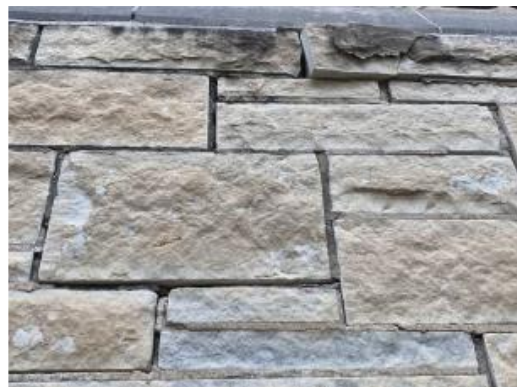
Displaced & loose stone
