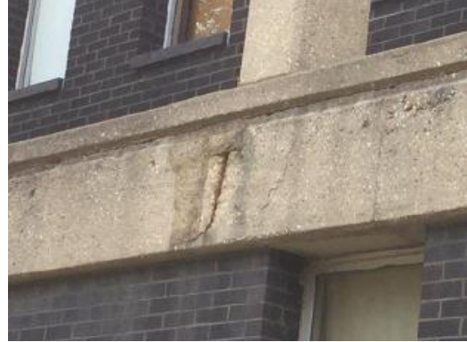
Exposed rebar
