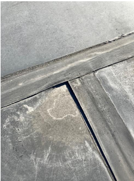
Roof seal separation
