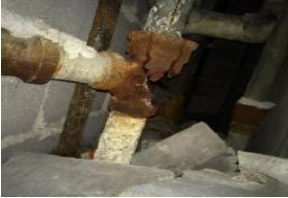
Corroded pipes
