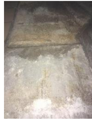
Water damage & efflorescence on limestone
