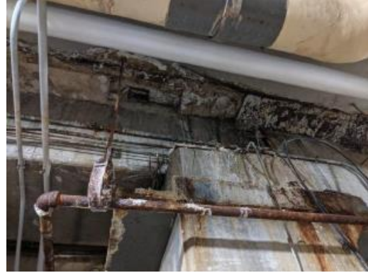
Corrosion from leak
