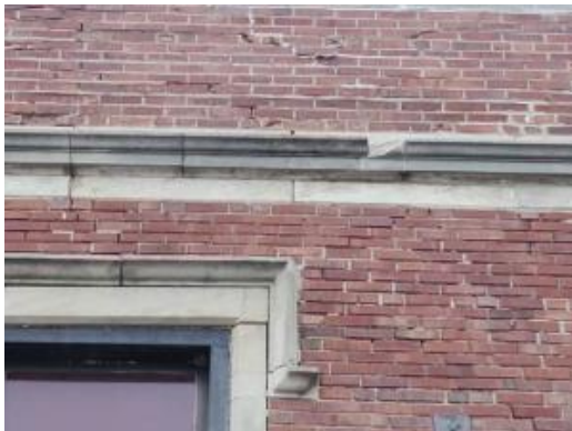
Spalling masonry and open joints
