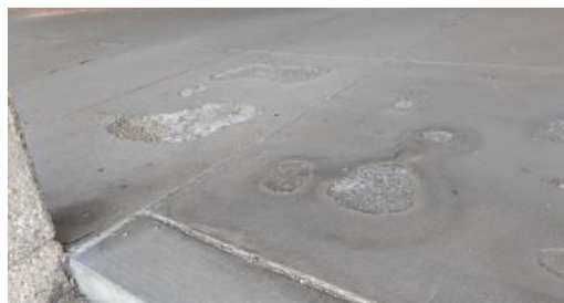
Spalling concrete floor
