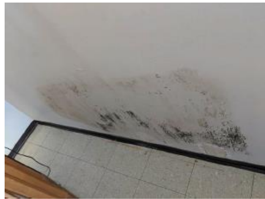
Mold from roof leak
