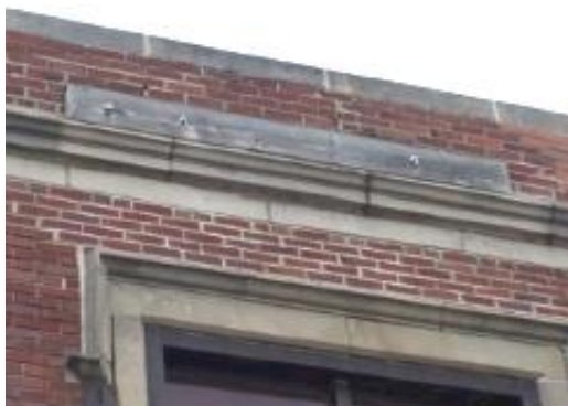
Temporary wall reinforcement
