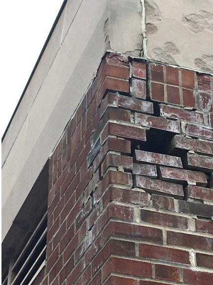
Masonry damage
