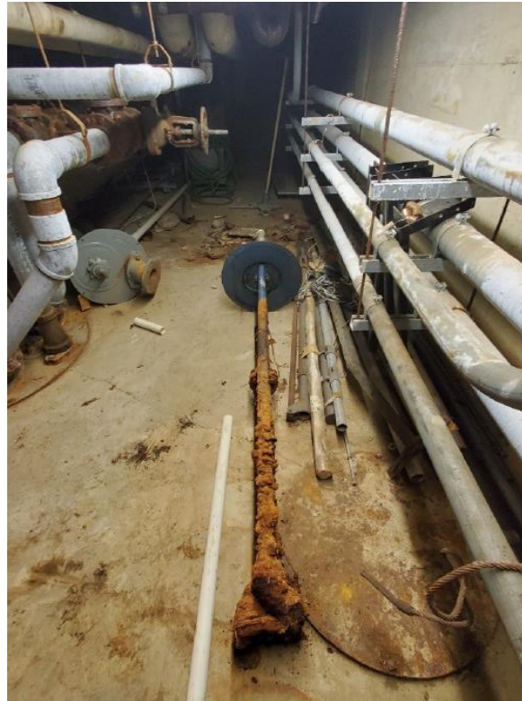
Sump pump scaling
