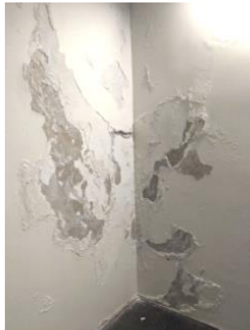
Drywall damage
