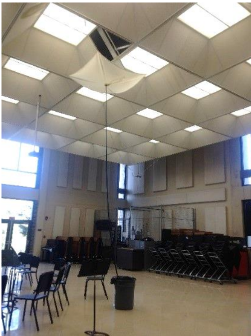
Ceiling leak (with improvised drainage system)
