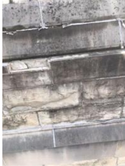
Displaced coping, fallen stone, 5" gap
