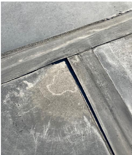
Aluminum cap damage & gasket popping out
