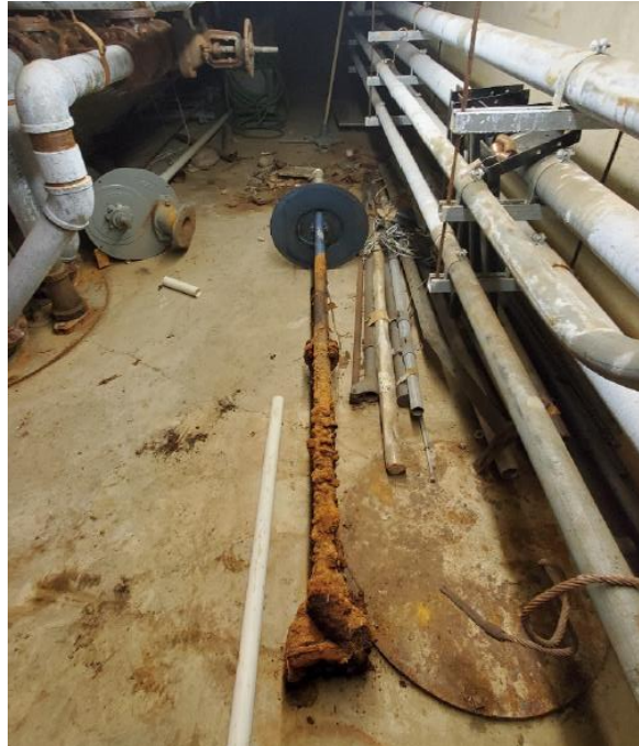
Corrosion from leak
