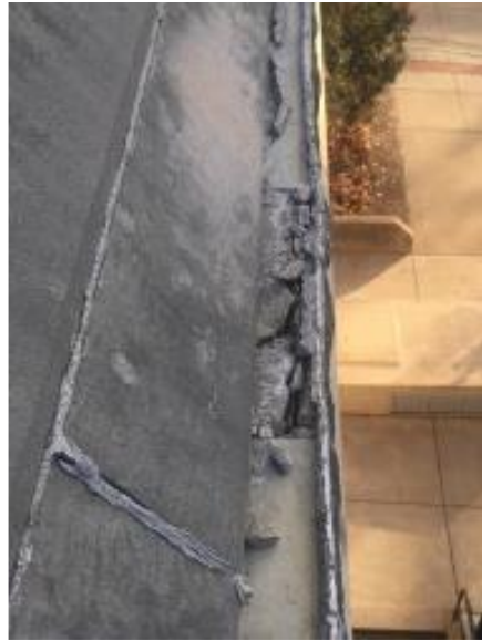
Displaced coping, damaged stone, wall exposed to elements
