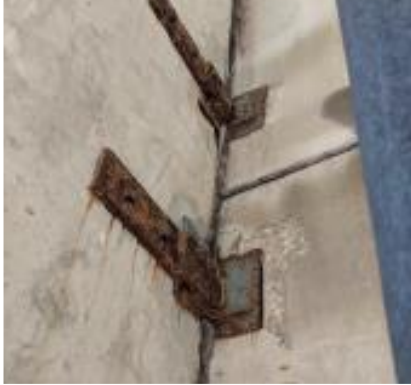
Rusted brackets, concrete pulling away
