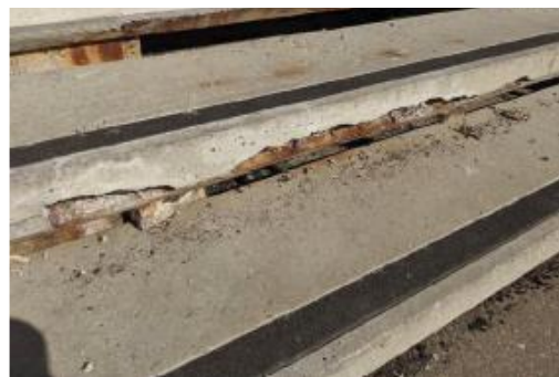
Damaged entry stair tread
