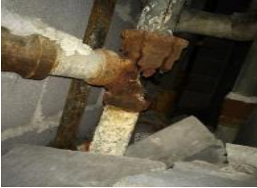
Corroded pipes
