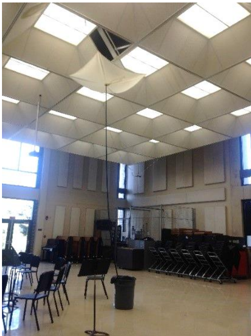
Ceiling leak (with improvised drainage system)
