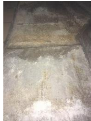
Water damage & efflorescence on limestone
