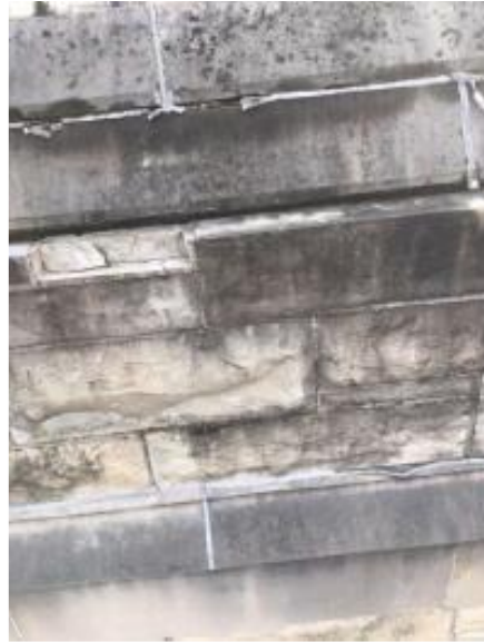
Displaced coping, fallen stone, 5" gap
