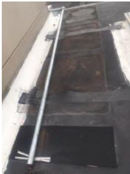
Deteriorating roof patches
