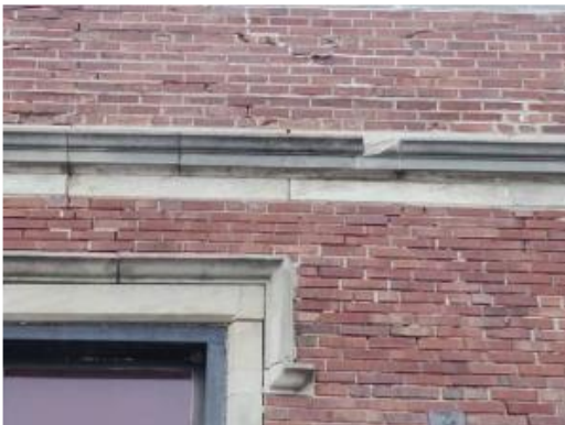
Spalling masonry and open joints
