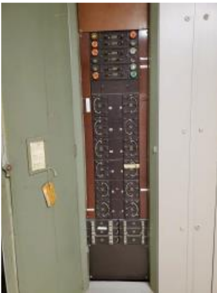
Antique screw-in fuse box (1940s)
