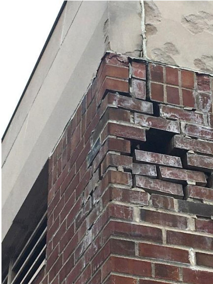
Masonry damage
