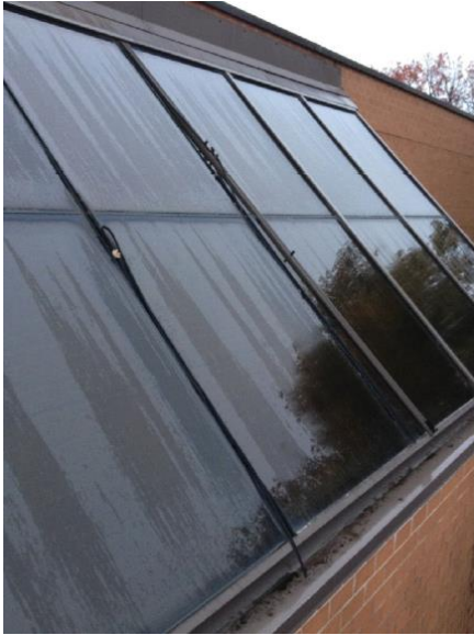
Aluminum cap damage & gasket popping out
