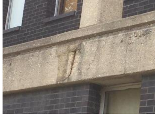
Exposed rebar
