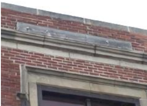
Temporary wall reinforcement
