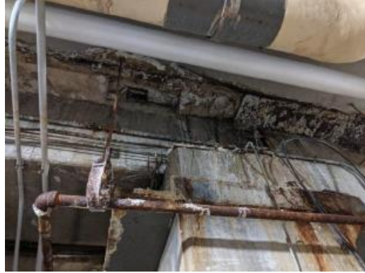
Corrosion from leak
