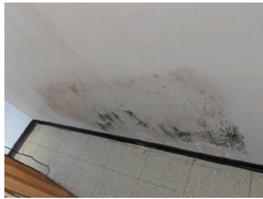
Mold from roof leak
