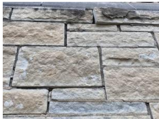
Displaced & loose stone
