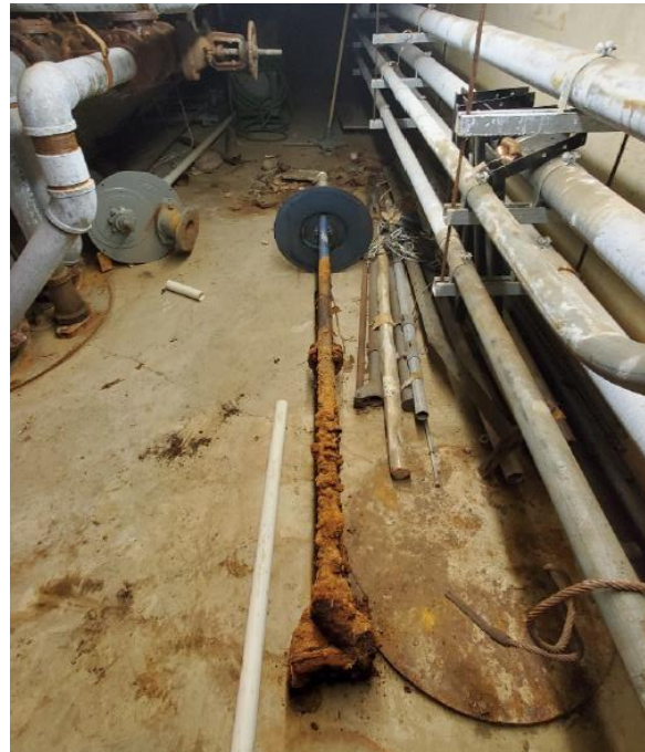
Corrosion from leak
