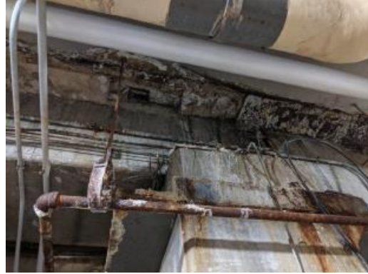
Corrosion from leak
