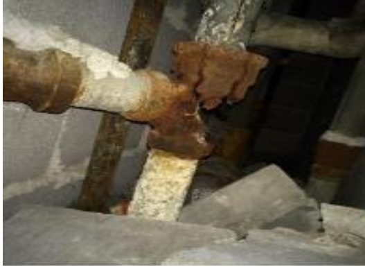
Corroded pipes
